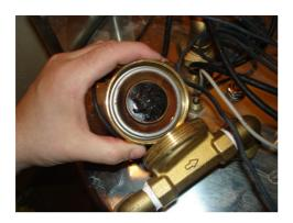
The rotor ball in the interior of the pump then becomes visible.
